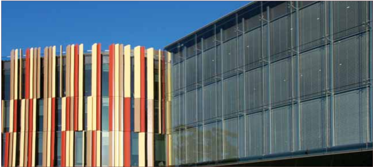
Retractable Horizontal Louvers - internal. University building.
