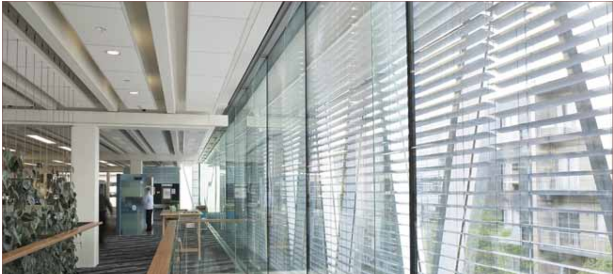
Retractable Horizontal Louvers - double skin facade. Insurance company headquarters.
